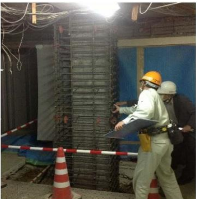
Jacketing of columns
