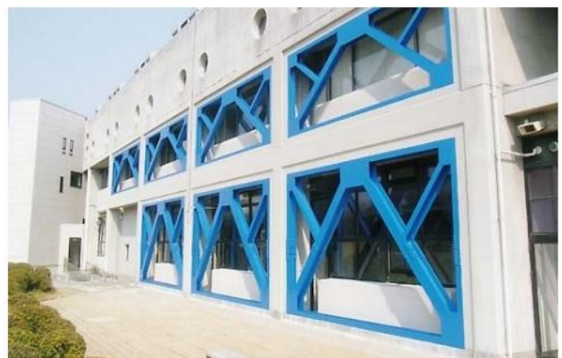
Additional steel braces
