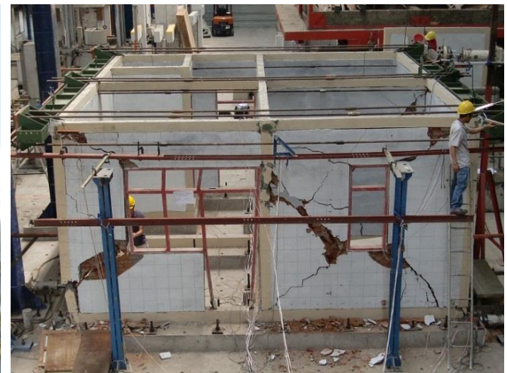
③ Full-scale structural test (governmental oversight improvement project)
