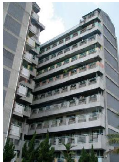
② Experimental housing (multiple dwelling optimum technology development project)
